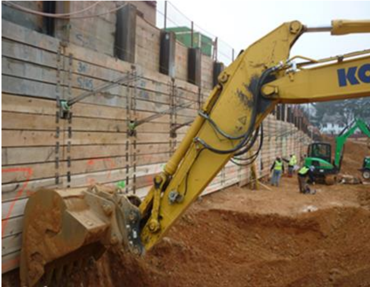
Excavation, Soldier Beams and Lagging
