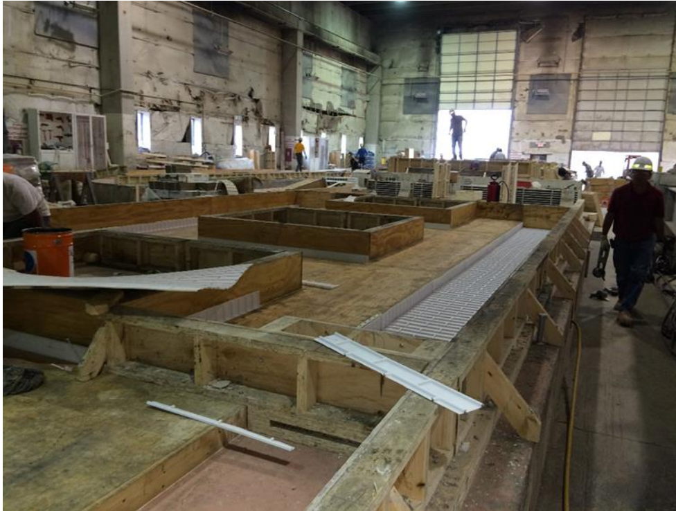
Façade prefabrication
