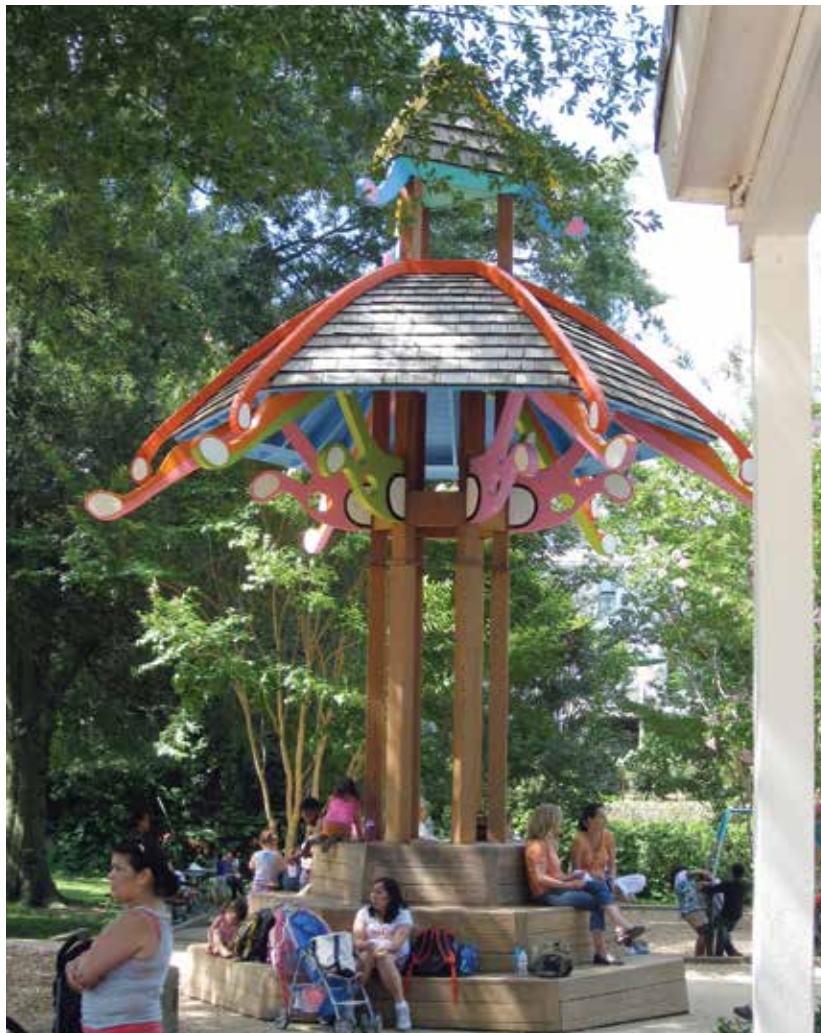
Macomb Street Playground Gazebo , 1981. Fir, cedar, glulam beams, steel frame, metal flashing, and latex enamel paint. Cleveland Park, Washington, DC. (Pete Ganginis, contractor)
