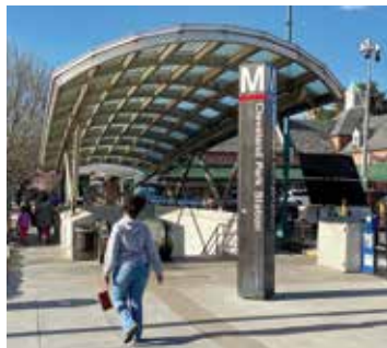
Existing Cleveland Park Metro canopy.
