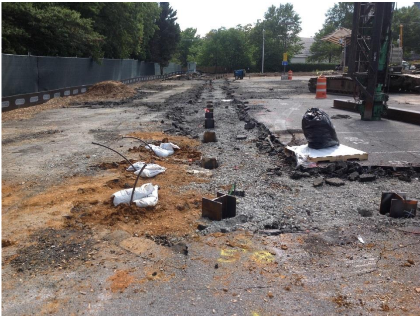
Soldier Pile installation
